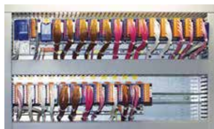
PCD3 in multiple-row mounting in the switch cabinet
