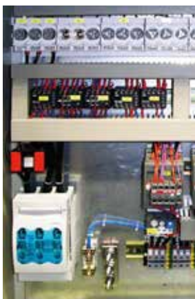
▲ Current converter in switch cabinet
